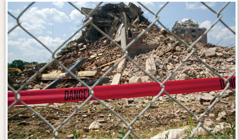
Detroit, Michigan — Demolition of the Brewster-Douglass public housing projects.
