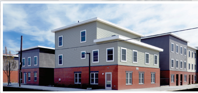
Grace Townhomes formed by the Community Justice Land Trust. Photo: Domus, Inc
