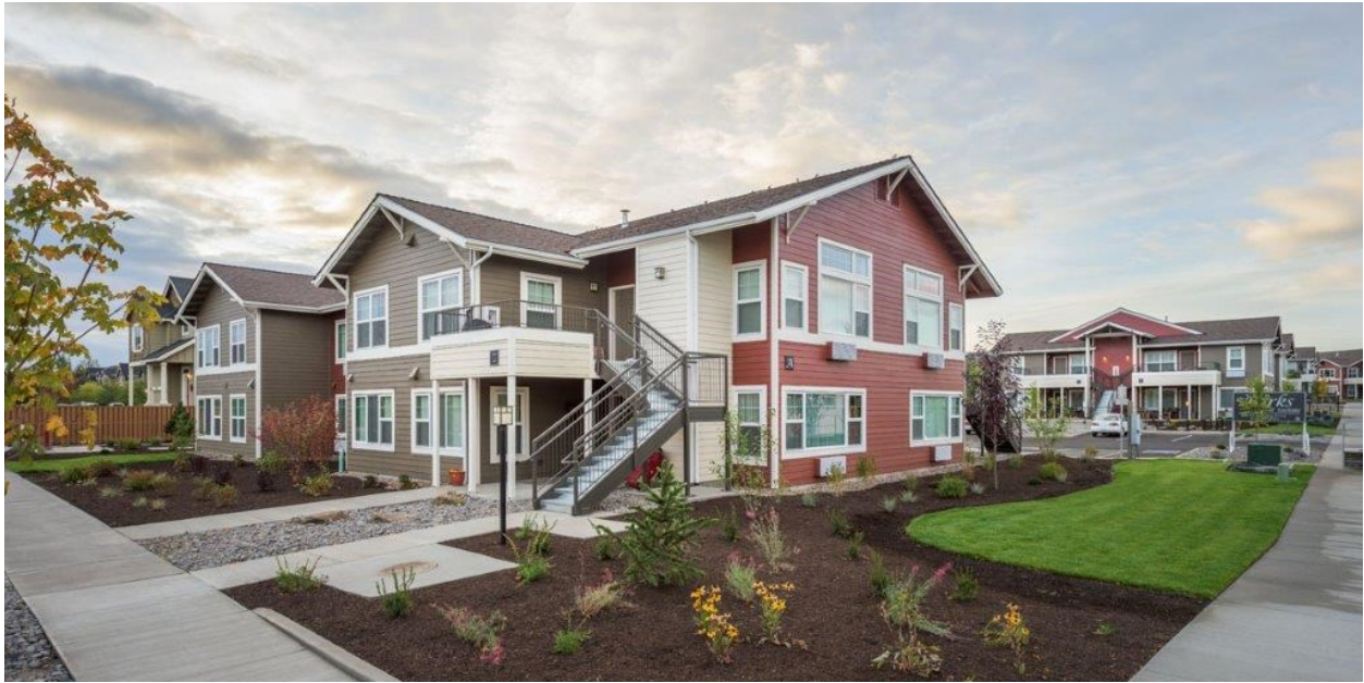
Project Name: The Parks at Eastlake and Aspen Villas Workforce housing Location: Bend Resource Funding: HOME and LIHTC Completed: 2016
