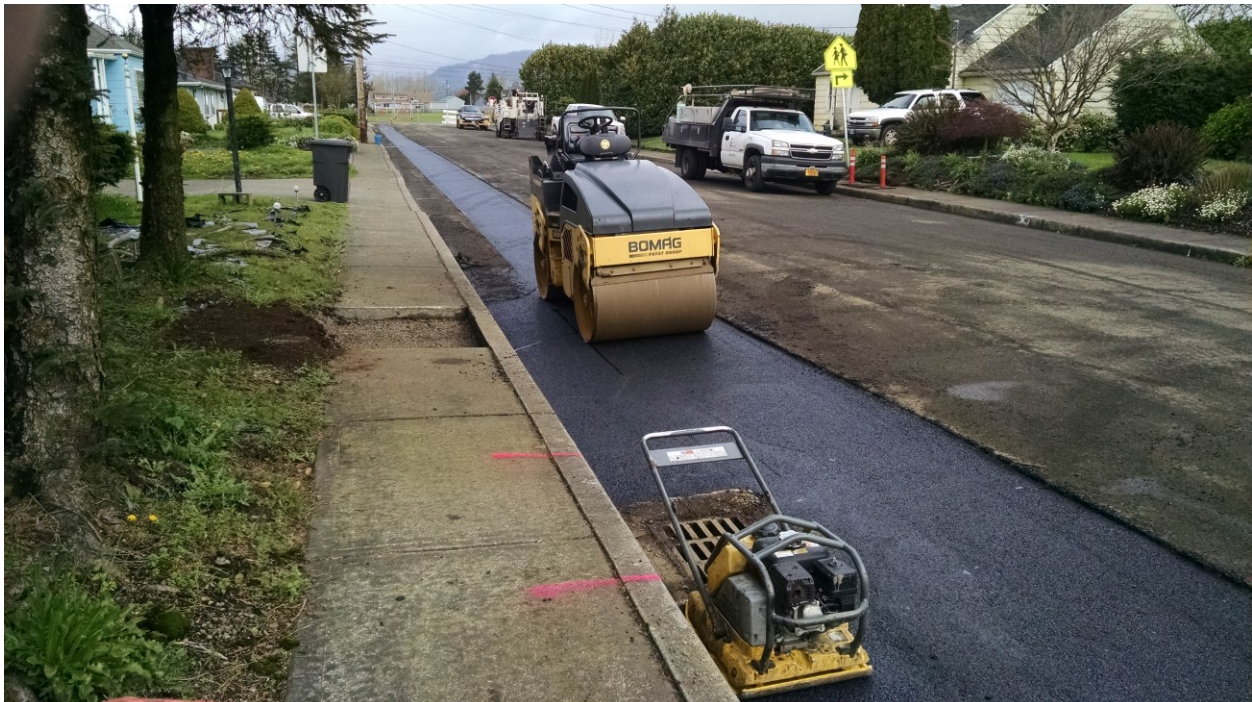
Project Name: City of Tillamook Collection System Improvements Location: Tillamook Resource Funding: CDBG Completed: 2016
