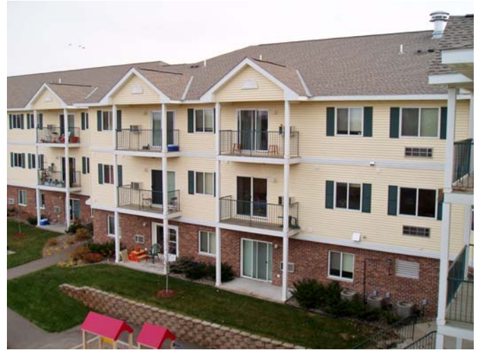
Multi-family apartment building in Scott County
