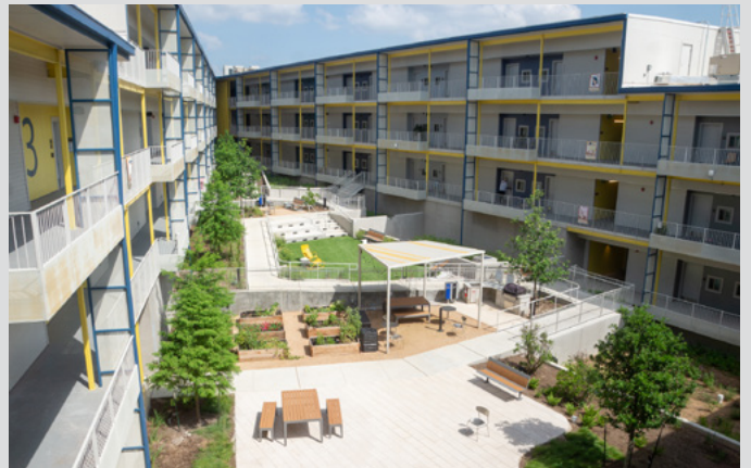
Waterloo Terrace, Foundation Communities Austin, Texas
