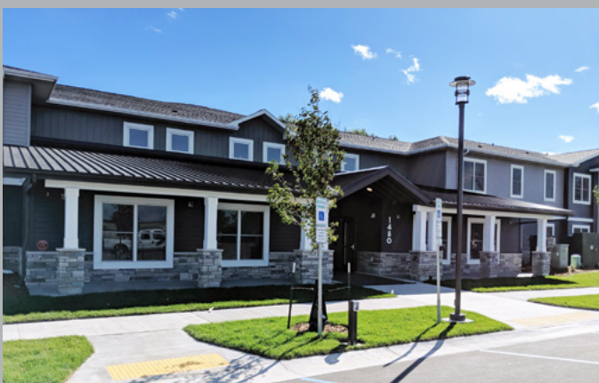
Grace Gardens, YWCA of Cass Clay, Shultz+Associates Housing for homeless women and children transitioning from domestic violence West Fargo, North Dakota
