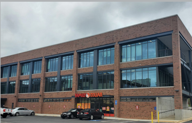
Holly Street Apartments Quest Community Development Organization Atlanta, Georgia
