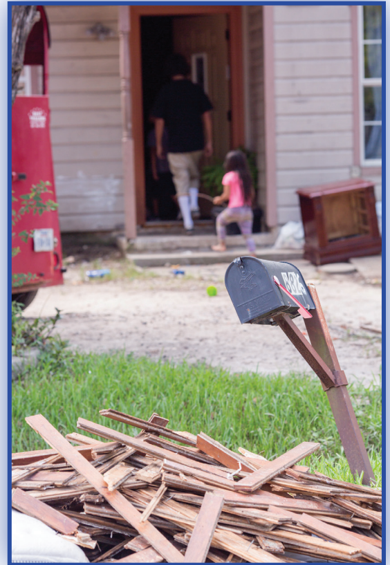
Flooding damage and recovery in the Lakewood Area of Houston, TX.
