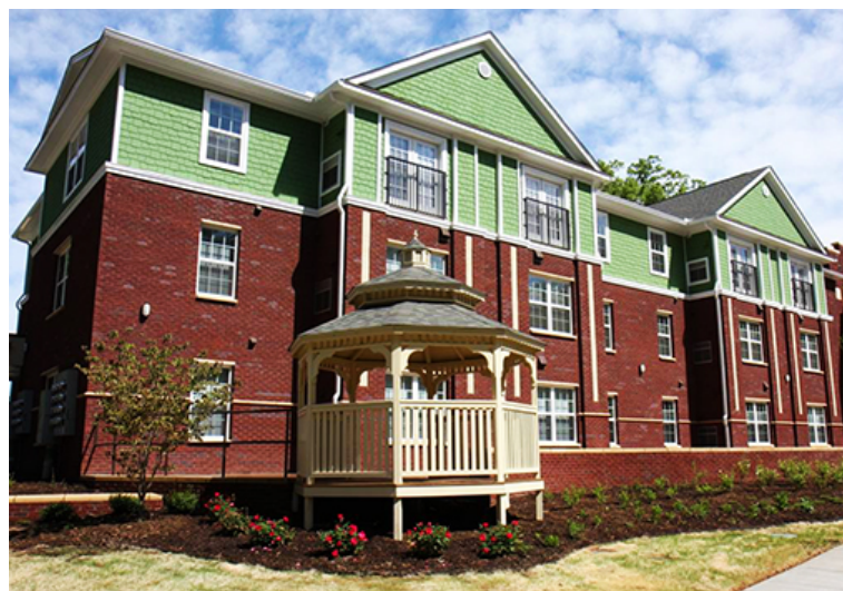
The Tyvola Apartments in Charlotte was funded through the Housing Trust Fund. It houses families between 30-80% AMI with a focus people with disabilities and people experiencing homelessness.
