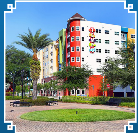
The Tempo at Encore, Tampa Housing Authority
