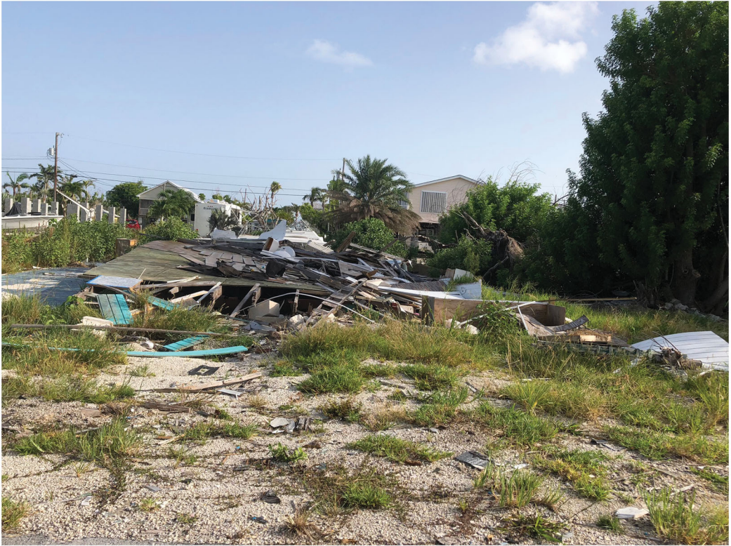
Figure 3. Hurricane damage in Big Pine Key, August 2018. Credit: Omur Damla Kuru.
