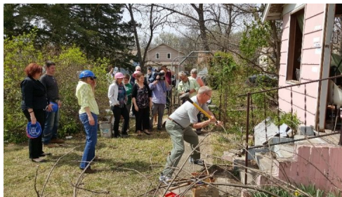
The success of the pilot project, shown here in the demolition phase, paved way for increasing investment in AHTF.
